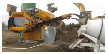
**Liquid soil:** When the soil-compound mixture is delivered, an appropriate amount of water is pumped into the truck mixer. The liquid soil is produced in batches and documented with a delivery paper. It is mixed in the truck mixer for 10-90 minutes and then poured.
