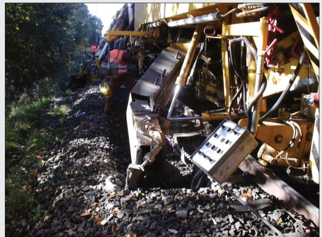
Removal of the contaminated railroad ballast from the railroad
