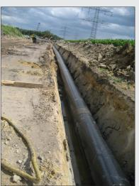
Direct backfilling of the screened fine grain into the pipe shaft
